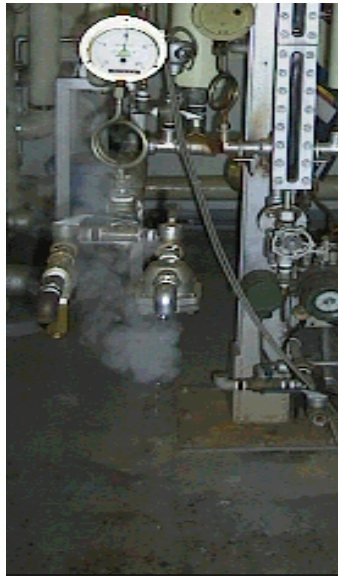
Free Float Steam Trap (Model: SS1N)
