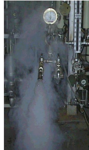
Fixed Orifice Steam Trap
